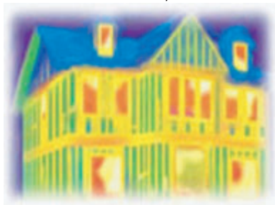
Roof insulation, no EIFS
